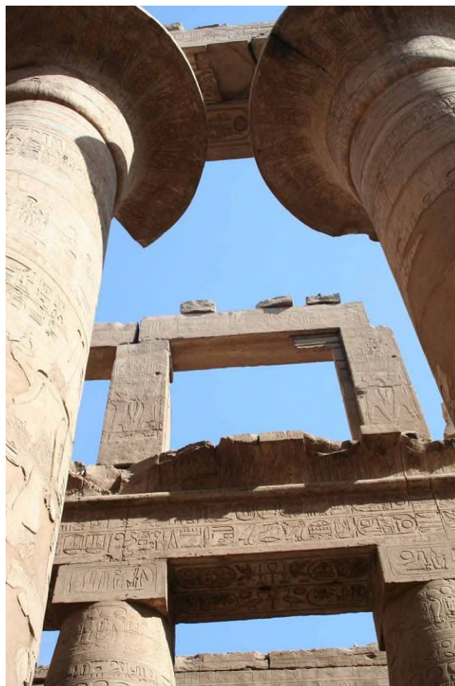
In the foreground the higher columns, in the background the capitals of the lower columns, with on top of the architrave one of the windows (now empty).
